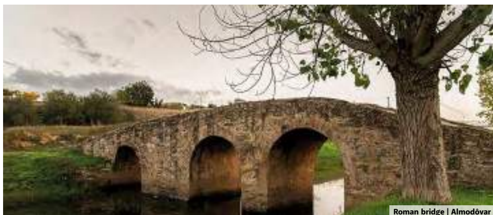
Roman bridge | Almodóvar
